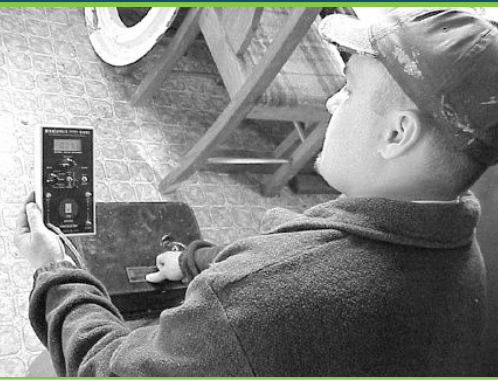
Delaware crews use a digital manometer to identify duct leakage.
