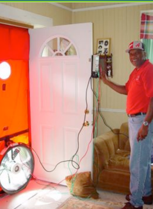
Blower door tests are conducted during the assessment of a weatherization home.
